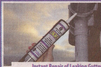
Instant Repair of Leaking Gutters
